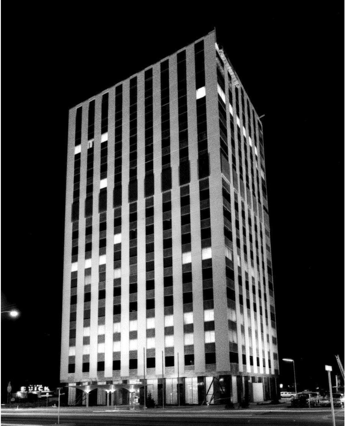
The First National Bank building at Central and San Mateo in 1963. The top two floors were an exclusive club. The bottom two floors were used for bank operations and open to the public. (Journal Archives)
